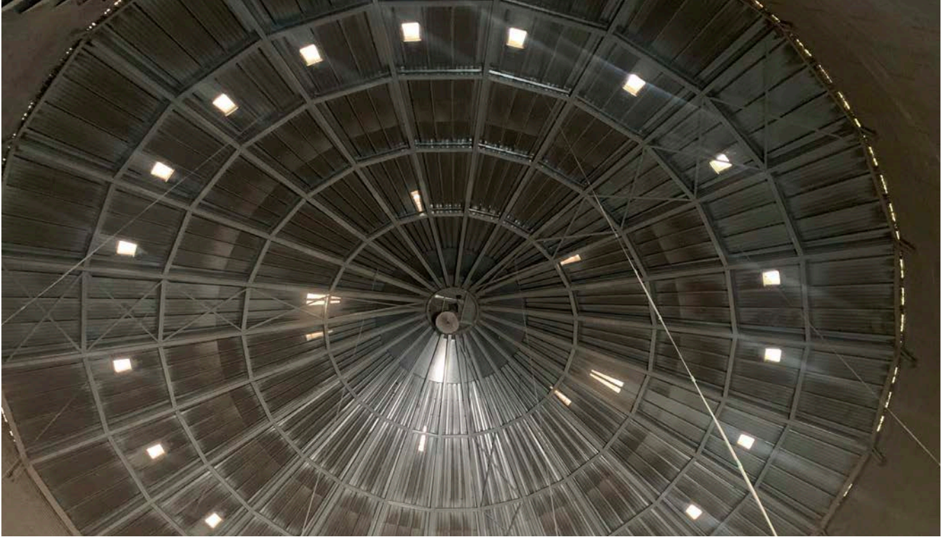
Image 11.4. Many larger grain bins have sensors on cables mounted on the roof to monitor grain temperature and moisture to help ensure the grain is storing properly.
