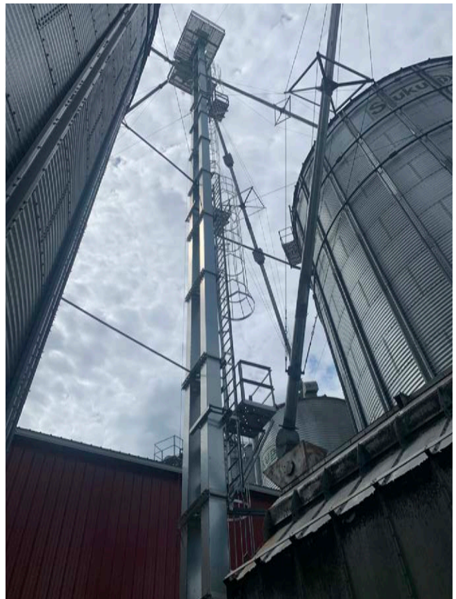
Image 11.5. Grain legs must be tall enough to provide proper angles to allow grain to fall into bins by gravity.
