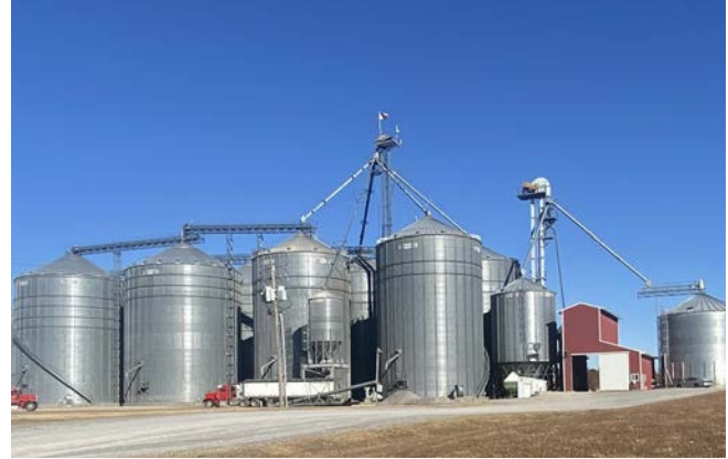
Image 11.2. Many on-farm systems include driers, wet bins, load-out bins and several storage bins.
